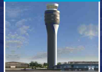
Sir Seewoosagar Ramgoolam International Airport, Mauritius (Under Construction)
